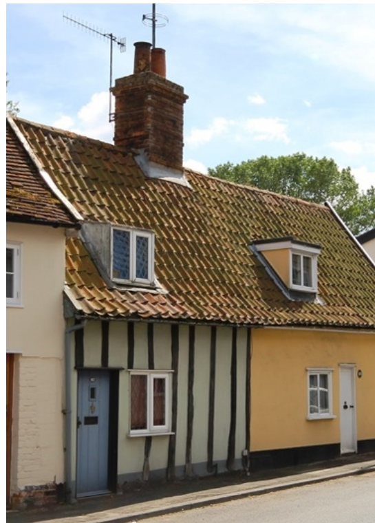
Exposed timber framing, Lower Road
