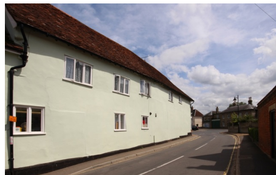
No.54 High Street, Broad Road elevation
