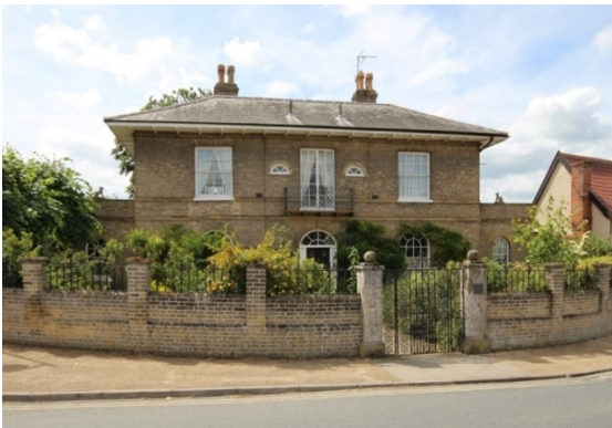
Hill House, No.52 High Street
