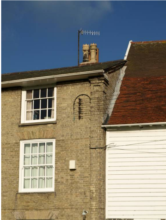
Pilaster detail, The Mill House, Deben Mills
