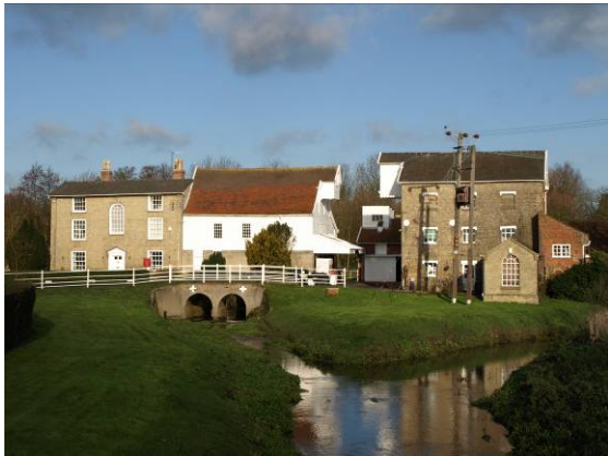
Deben Mills from the road bridge
