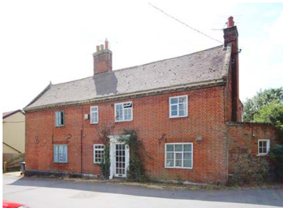
No.s 1-3 Mill Lane
