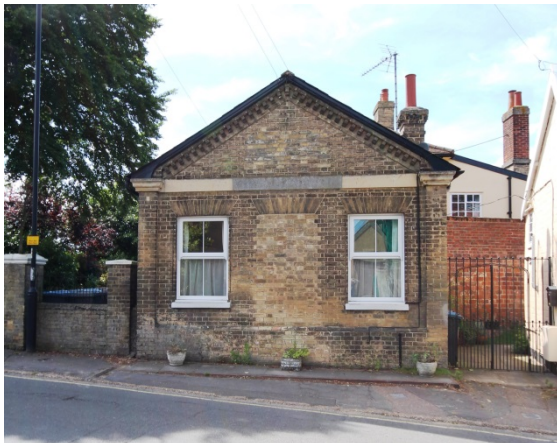
Former Post Office No. 80 High Street
